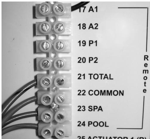
Figure 12. Heater Wiring Block — Analog Heaters
