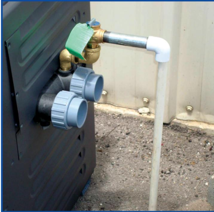
This photo illustrates the correct installation of a PRV on the larger models.
