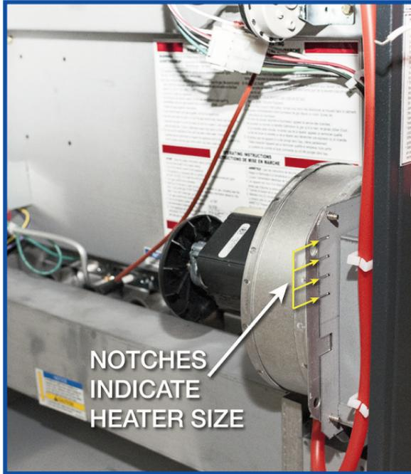
Notches Indicate Heater Model Size:
