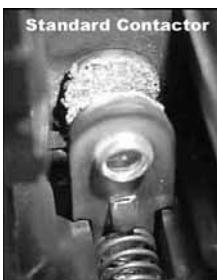
**contactor and features optical control and latching mechanism.** The sealed switch prevents infiltration of insects and dust. A minimal switching arc, by the optical control, offers greater reliability. The latching mechanism consumes less power while reducing chatter.
